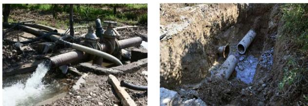
*Fig. 2 Damaged pipelines*
