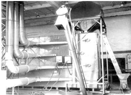
Fig 1. General view of the conveyor system for combined drying grain using microwave energy
