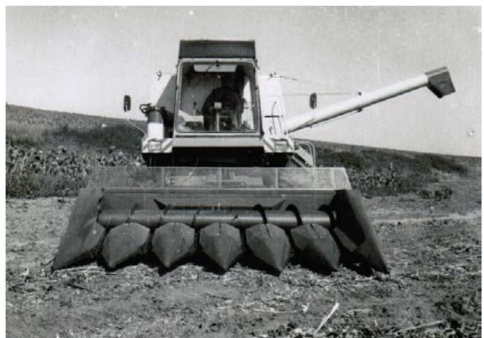
**Fig. 1** Row header for harvesting soybeans HPS
