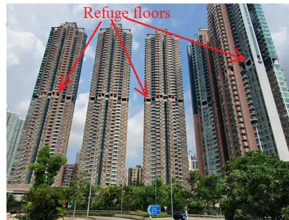
Fig. 5 Refuge floors in tall buildings in Hong Kong (Picture made by the author M. Ivanov in 2019)
