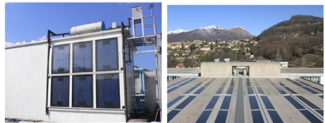
Fig.5. BIPV / T water system integrated in the facade of the building [16], BIPV / T roof system [17]
