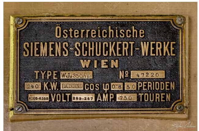
Fig. 3 Nameplate of one of the operating generators.
