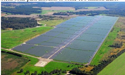
Fig. 10: Waldpolonez Solar Park built in on military air base to the east of Leipzig (Germany) [25, 33]
