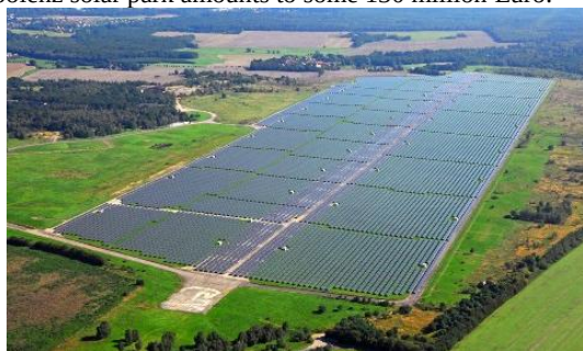
Fig. 10: Waldpolenz Solar Park built in on military air base to the east of Leipzig (Germany) [25, 33]
