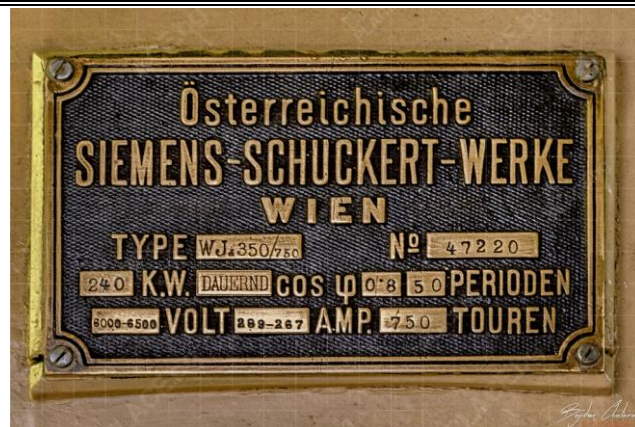
Fig. 3 Nameplate of one of the operating generators.
