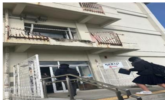
Fig. 2 Exterior wall of Arahama Elementary School
