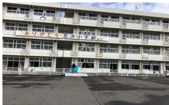
Fig. 1 Arahama Elementary School
