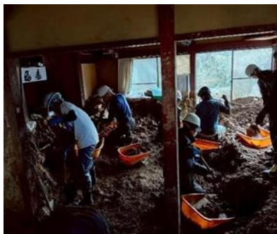
Fig. 4 Removal of soil and debris from inside a house.
