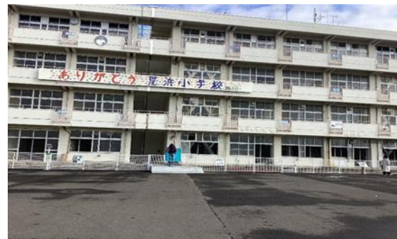
Fig. 1 Arahama Elementary School
