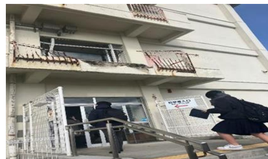
Fig. 2 Exterior wall of Arahama Elementary School
