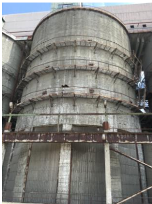
Photo 1 Silo's concrete structures visualization
