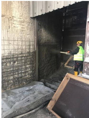
Photo 2 WS mix wet site-shotcreting
