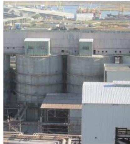
Photo 1 - Silos for Light Soda, SOLVAY town of Devnya, Bulgaria
