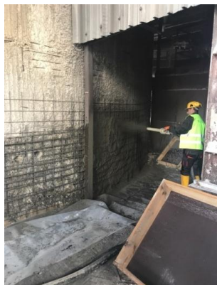
Photo 9 "Wet" WS spraying
