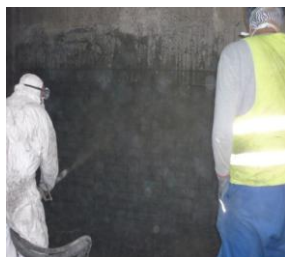
Photo 8 MC Torkret W81 spraying
