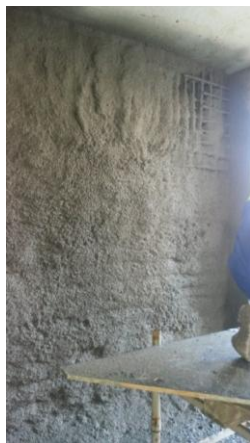
Photo 7 "Wet" shotcreted wall
