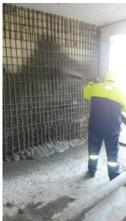
Photo 5 Shotcreting process
