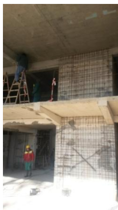
Photo 3 Supporting wall prepared for shotcreting
