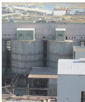
Photo 1 LIGHT SODA SILOS "4" & "5" general view
