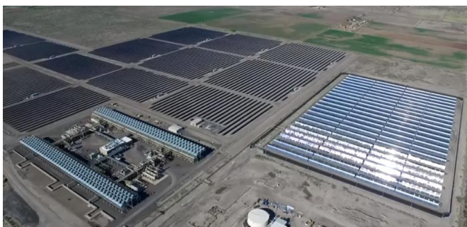
Fig. 1. Aerial view of the Stillwater triple hybrid geothermal-solar power plant, Nevada, USA.
