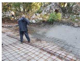
Photo 20 Wall spraying
