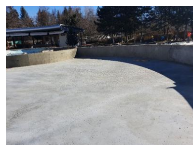
Photo 18 View of finished concrete works
