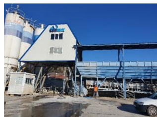
Photo 11 ECOMIX concrete batching plant
