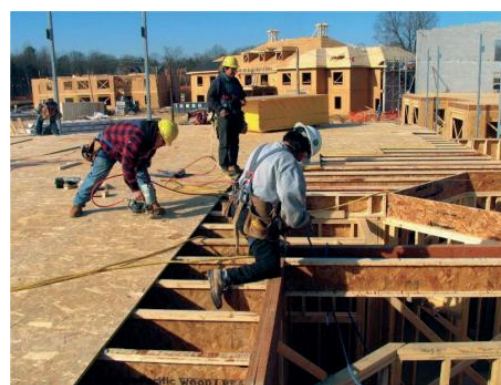
Figure 5. Flooring application of OSB panel.
