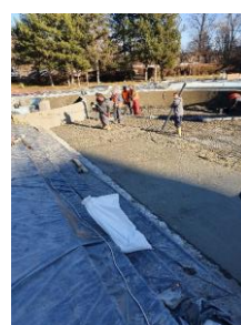
Photo 17 Bottom slab concrete casting
