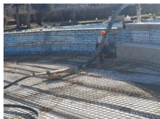
Photo 12 Walls and bottom slab steel mesh fixing
