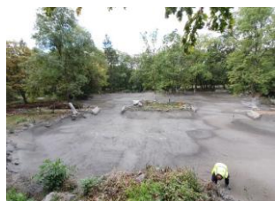
Photo 22 Finished area – walls and bottom slab
