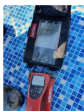
Photo 10 Direct scanning existing steel reinforcement - visualization
