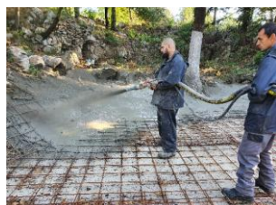
Photo 21 Wall spraying
