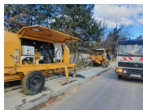
Photo 13 Concrete pumps used
