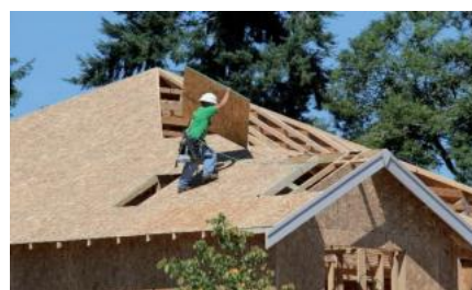
Figure 6: Roof application of OSB panel (Fig. 6).
