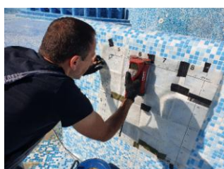
Photo 9 Direct scanning existing steel reinforcement
