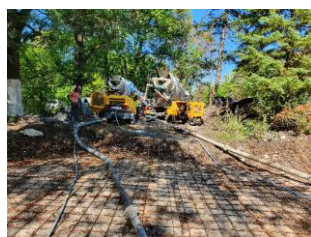
Photo 19 Deployment of two concrete pumps for simultaneous operation
