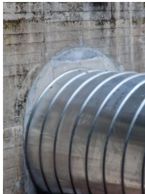
Photo 17 Tunnel 1 contour completed
