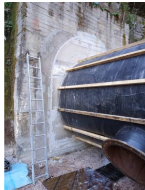
Photo 18 Tunnel 2 contour completed
