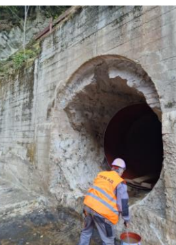
Photo 11 Tunnel 1 – preparing for formwork
