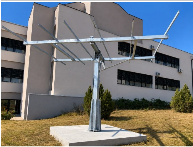
Fig. 16 Structural frame assembly
