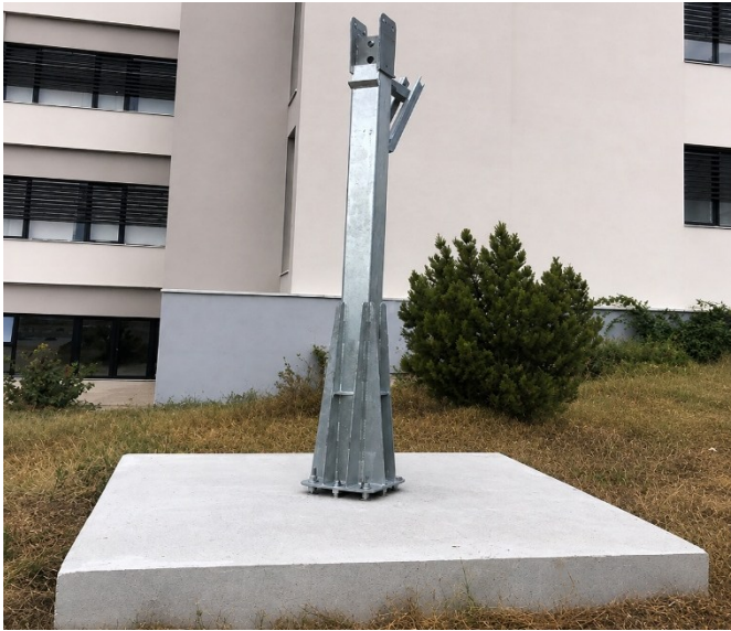
Fig. 15 Concrete foundation and installing vertical steel pole
