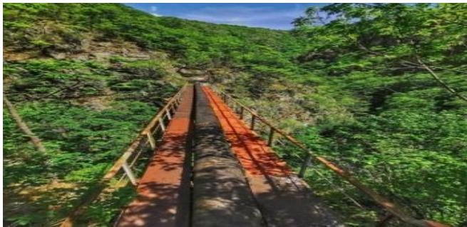
Fig. 2 Pressure pipeline of Tazha HPP.
