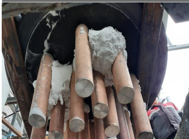
Fig. 1. Filter elements removal from reactor discharge unit
