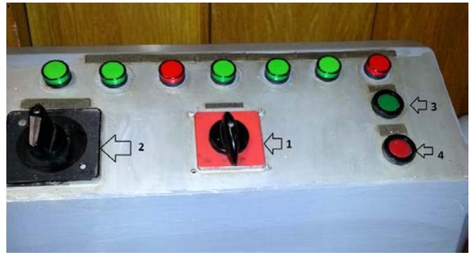
**Fig. 5** Burner control panel
