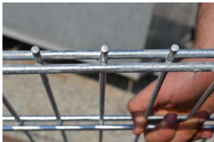
Figure 7 Bed welding spot
