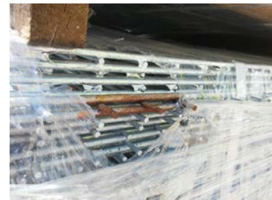
Figure 3 Corrosion attack on the coated bars
