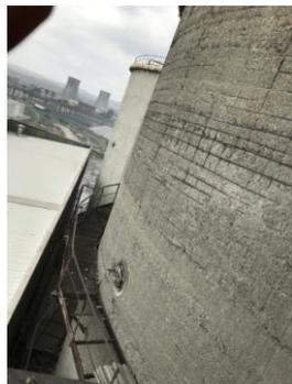
Photo 2 LIGHT SODA SILOS "4" & "5" typical concrete damages
