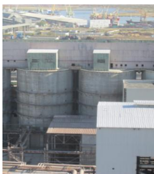
Photo 1 LIGHT SODA SILOS "4" & "5" general view
