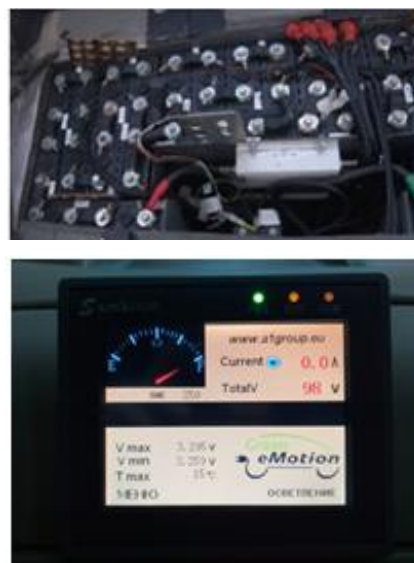
Fig. 1 The battery pack and BMS information display.
