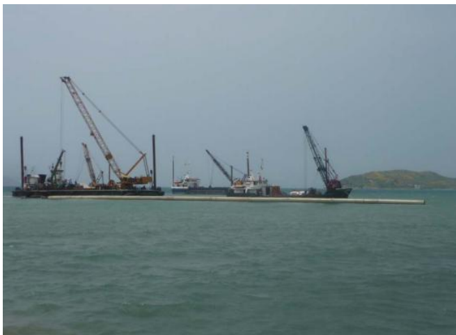
Figure 15. Floating of the pipe string DN 1600
