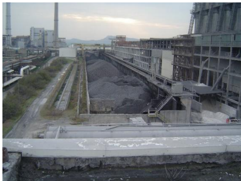
Photo 1 Open fuel storage – general view
