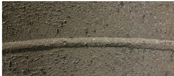
Fig. 9 Detail of the boiled root cutout from pipe No. 1
