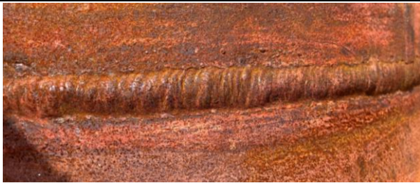
Fig. 8 Visual inspection of the weld surface – pipe No. 1
