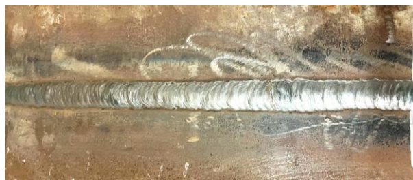
Fig. 10 Visual inspection of the new hot water pipe No. 2
