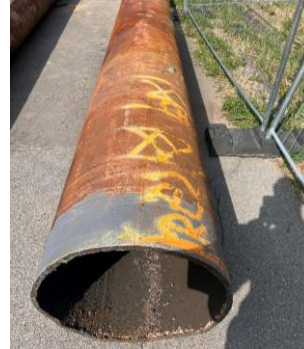
Fig. 1 Cutting of pipe No. 1 from the original hot water pipe
