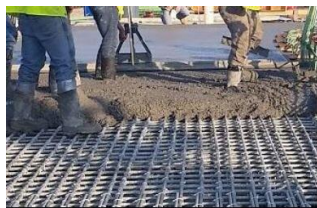
Fig. 1 GFRP reinforcing bars used in a concrete slab
