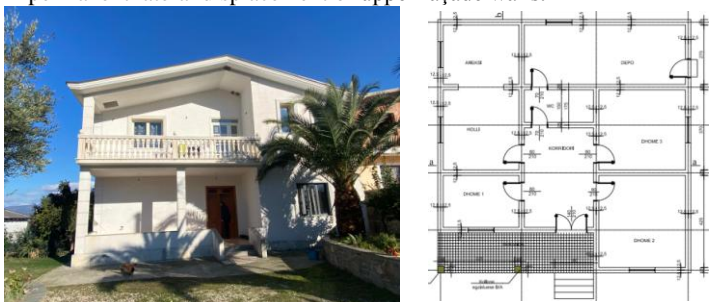
Fig. 4 Building façade photos (right), plan view (left).
