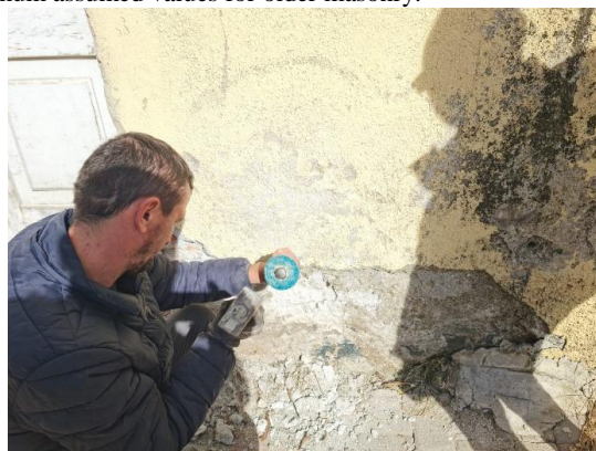
Fig. 7 Testing sample extracting Building 2.
