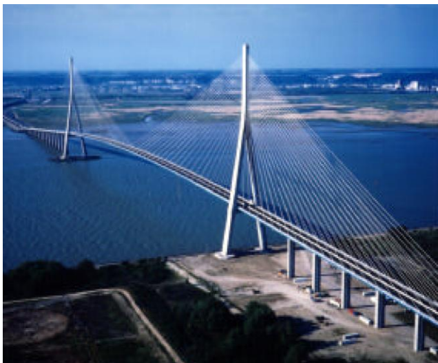
Fig. 1. Normandia bridge – example for a large cable-stayed bridge [8]
