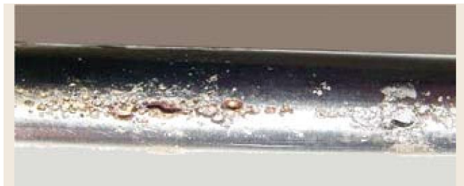
Fig. 5 Pitting corrosion of the tubing [10]
